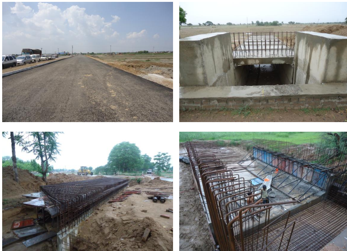
Photo 3.1 Photographs of construction of Rohtak-Bawal NH
